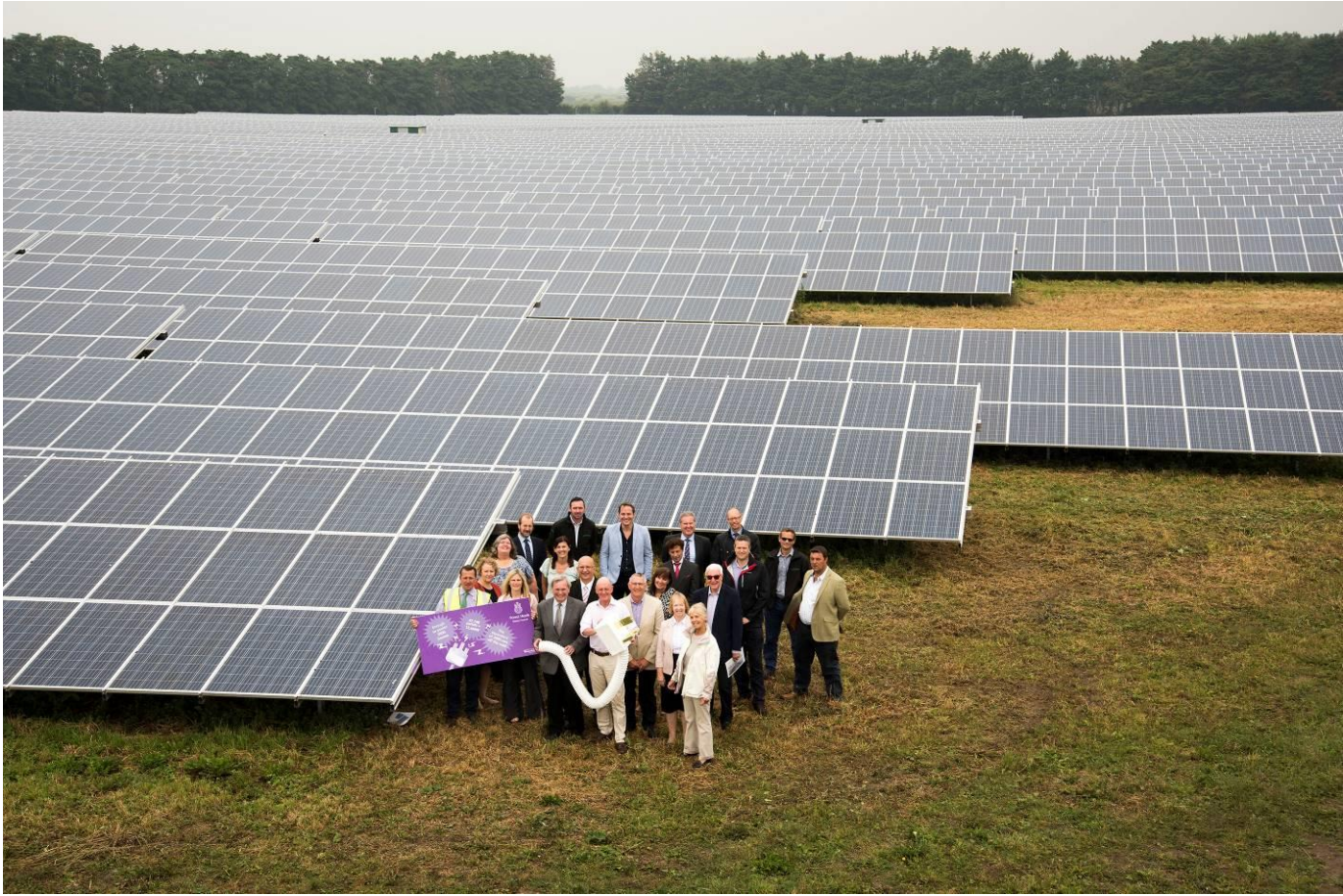
Solar Farm, Lakenheath
